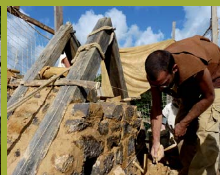
The masonry on the gable's interior wall nears the end.
