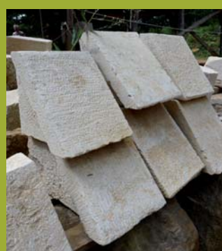
The copings ready to be laid.
