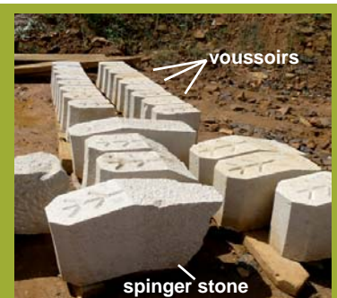
Springer stones are much longer than the voussoirs
