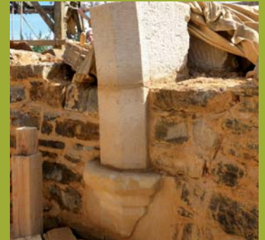
The corbels and nearly all the springers are in position.
