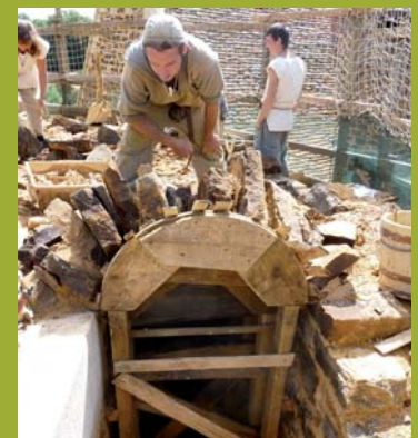
Barrel vaulting under construction.
