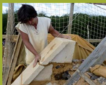
The last copings are laid.
