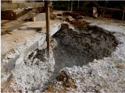
The base of the corner tower is filled with lime putty
