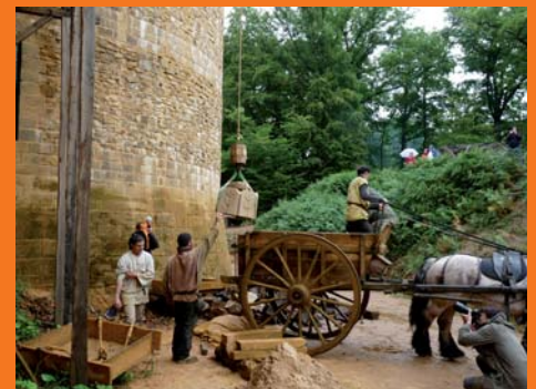
The keystone is hoisted up onto the tower
