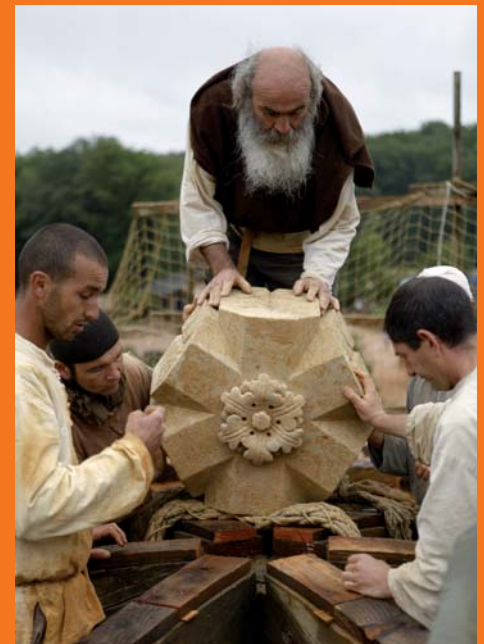
The keystone is gently positioned on the centring
