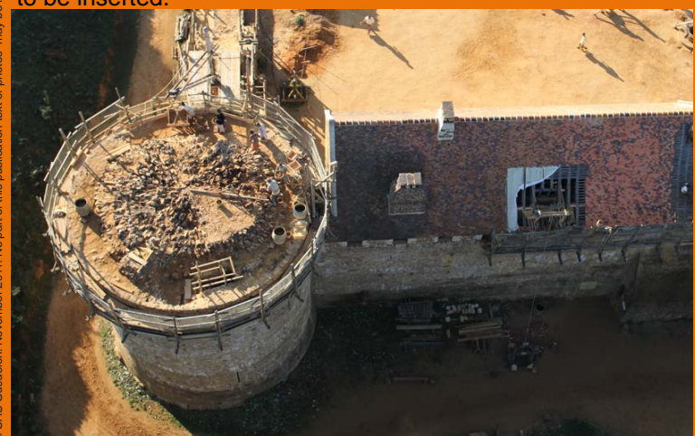
14 October 2011: the webbing is complete and the vault is under load.
