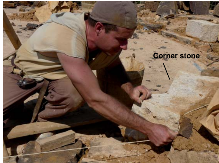
Fixing and adjusting one of the octagonal chamber's corner
