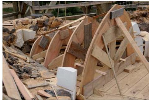
The masons have positioned the 4 formers: wooden supports in the shape of the vault. On these formers, they will then lay wooden shuttering. This forms the wooden structure which will support the masonry of the vault.
