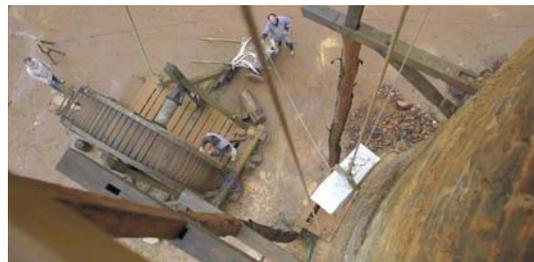
The final corbel was hoisted on to the tower by the treadwheel winch. It was then moved into position on wooden rollers. This was a difficult operation due to the weight of the stone and the delicate floral sculpture on the corbel's outer face. The corbel weighed in the region of 150 kg.
