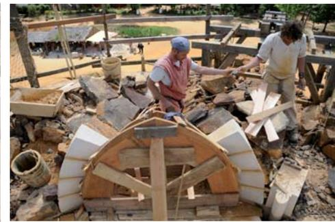
The first 4 limestone voussoirs, on each side of the pointed arch have been fixed. The masons then install the shuttering, followed by edge-bedded sandstone flagstones.
