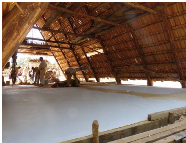
Fabrice using a mason's level during the paving of the Great Hall
