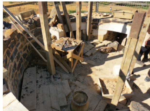
1: curved wall plates 2: straight wall plate of the cut-off inner wall 3: roof timbers stocked in the workshop
