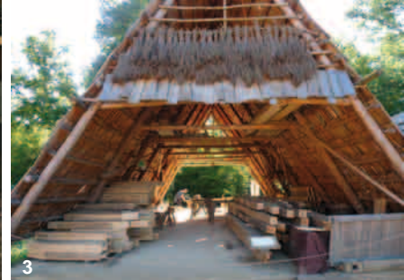
1: curved wall plates 2: straight wall plate of the cut-off inner wall 3: roof timbers stocked in the workshop
